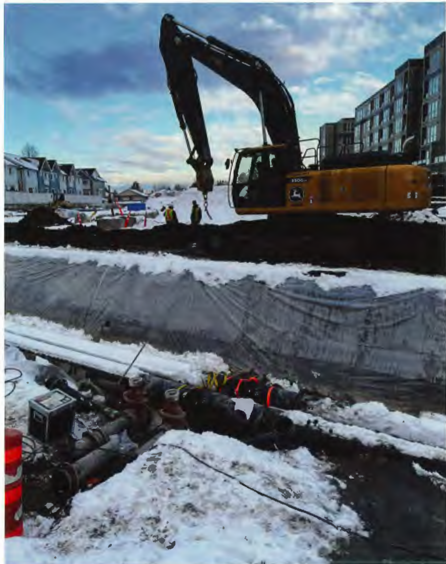
Implementing distribution piping in the ADEU.
