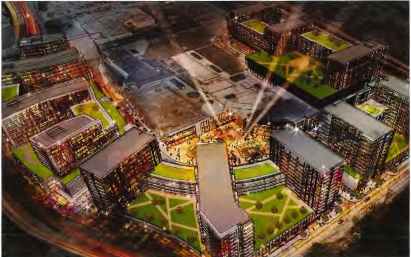
The Richmond Centre development currently under construction.
