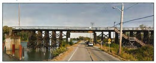
The existing maximum road clearance below the structure is posted at 5.88 m. Raising the road/dike would reduce the clearance.
