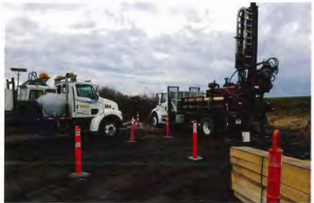
Microbial Induced Desaturation and Precipitation Test
