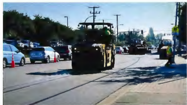
High Recycled Asphalt Pavement Project
