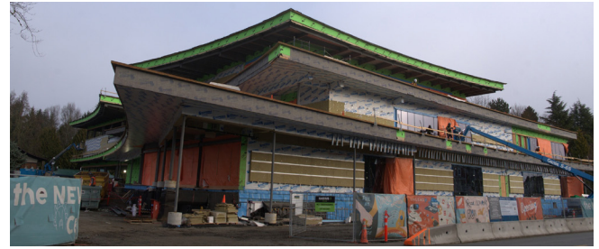
Steveston Community Centre and Library Construction
