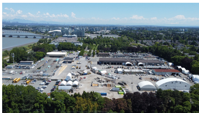
Major Construction Project – Works Yard Replacement Project
