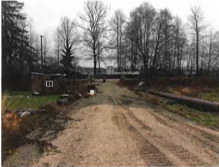
PHOTO 3: NEW GRAVEL DRIVEWAY (AND CROSSING IN BACKGROUND TO THE CENTRE) THAT CONNECTS THE PROPERTY TO RIVER ROAD. THE DRIVEWAY HAS BEEN BUILT ABOVE THE NATURAL GRADE BY UP TO 0.5 M ACCORDING TO THE LAND SURVEY.
