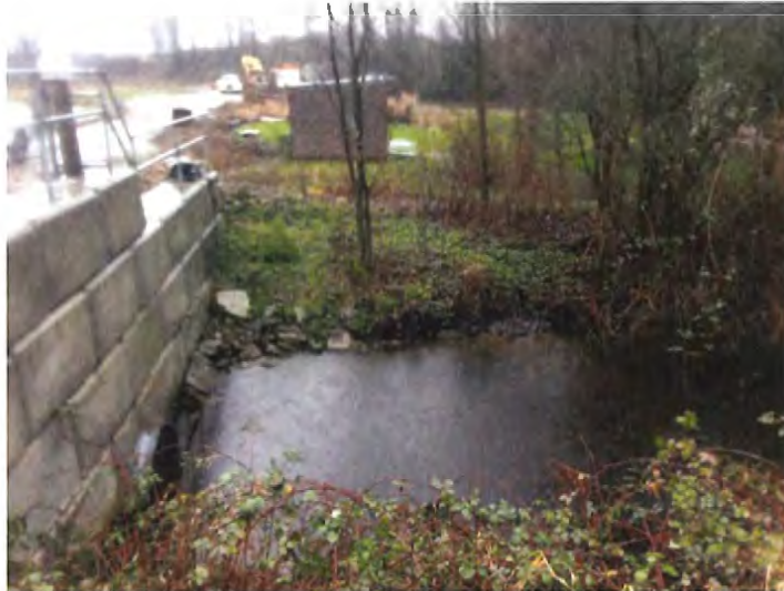
PHOTO 12: LOOKING DUE SOUTH ACROSS THE ENTRANCE OF 17260 RIVER ROAD. THE SOIL PLACEMENT AREA IS LOCATED IN THE TOP LEFT CORNER OF THE PHOTO. THIS CROSSING WAS UPGRADED IN 2019 - THE OLD CROSSING WAS SITUATED TO THE RIGHT OF THIS PHOTO.
