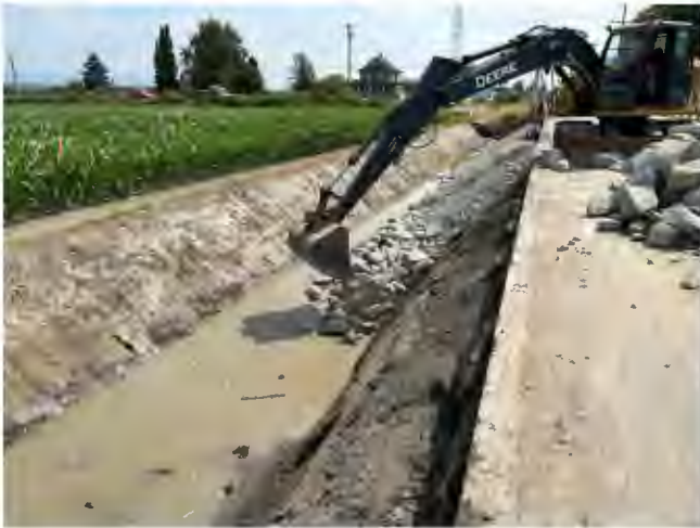
Canal Stabilization Works
