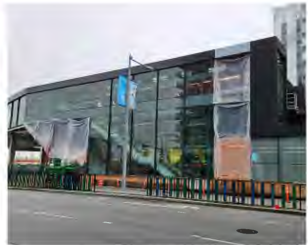
Capstan Station Construction
