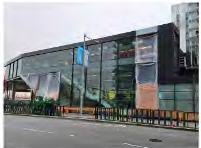
Capstan Station Construction
