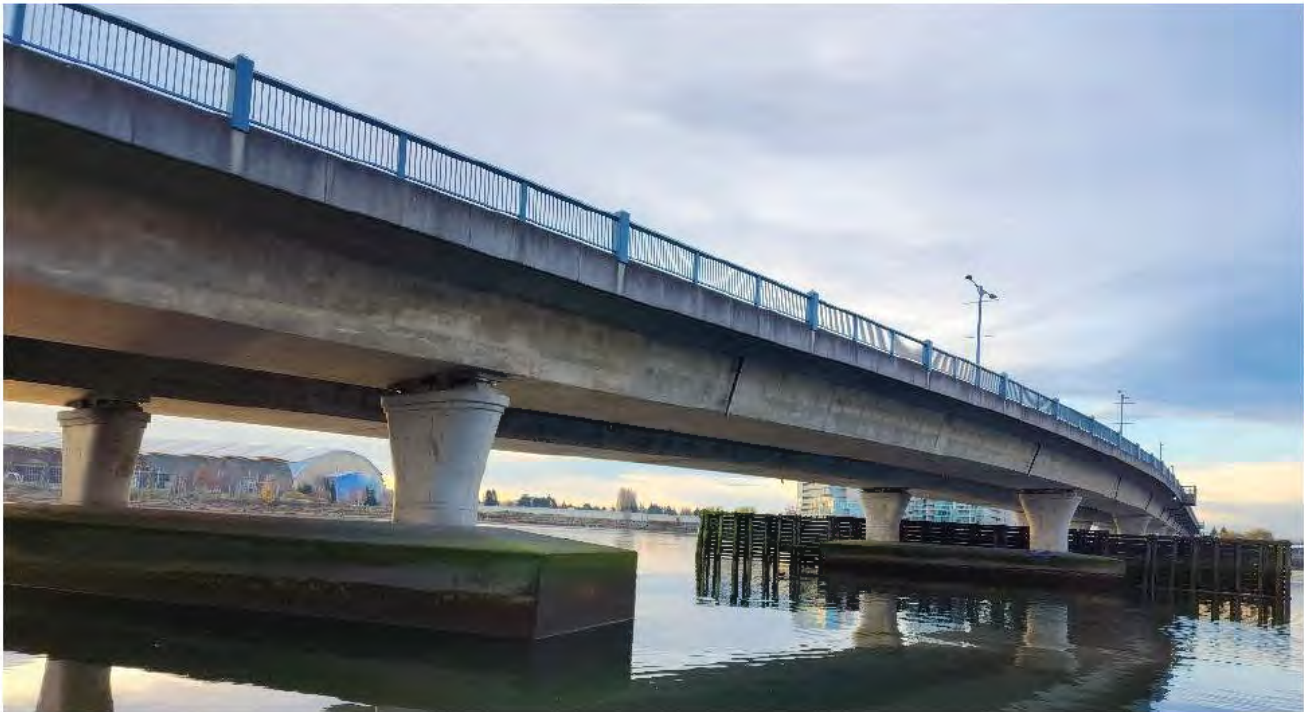
Bridge Condition Assessment
