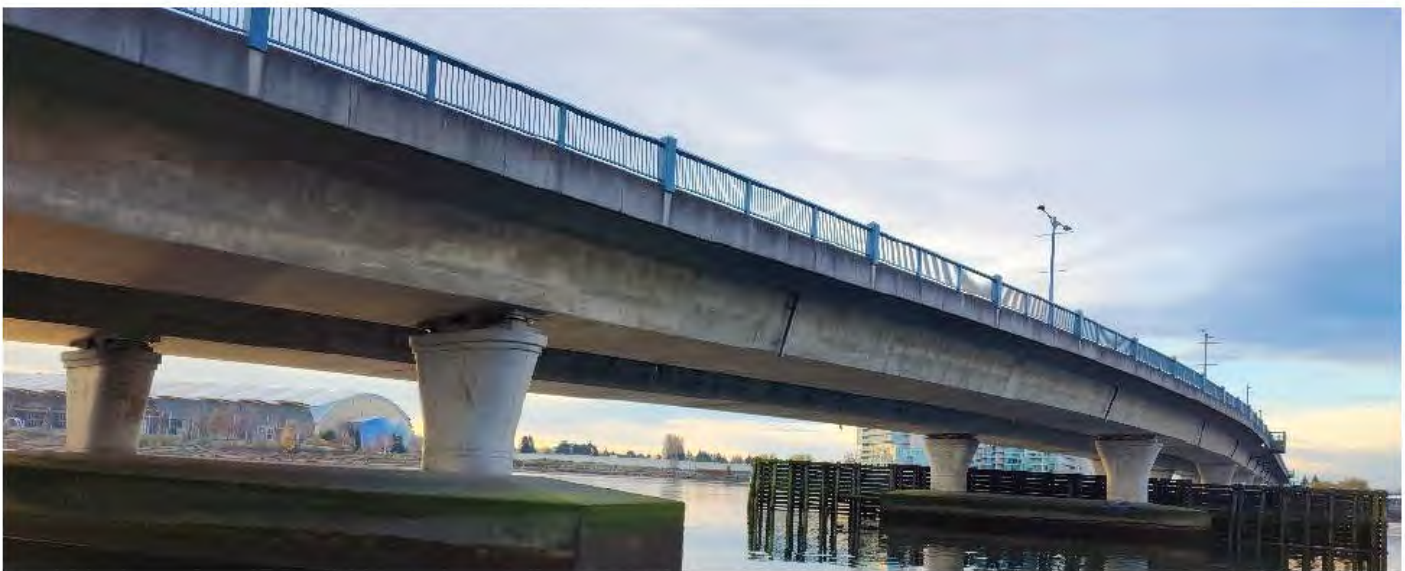
Bridge Condition Assessment
