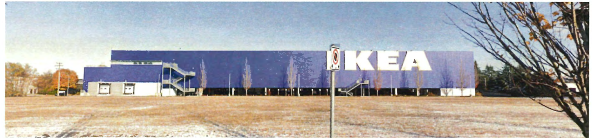
2 Existing South View (Photos taken from Google Earth)
