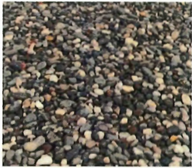
EPDM ROOF MEMBRANE ROCK BALLAST
