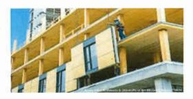
A building system using Encapsulated Mass Timber is flexible, working in conjunction with other materials and systems. Typically, the elevator core may be constructed of reinforced concrete while the building envelope may be of any suitable material or design. In the Brock Commons example, the building skin comprises a pre-manufactured assembly of metal, wood, glass and insulation installed on site.
