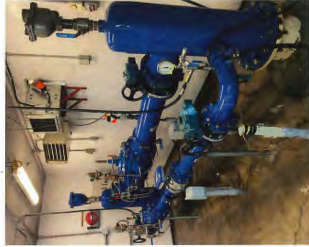
A look inside a pressure-reducing valve station.
