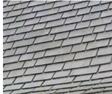
NEW TREATED CEDAR SHINGLE ROOF IMAGE
