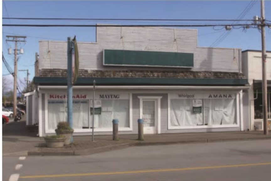
Figure 26: Storefront windows and single door with shingled canopy and older signage attached, 2022.
