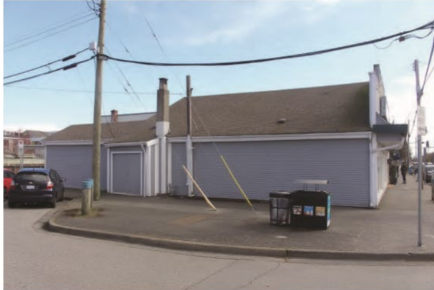
Figure 33: West side of subject site, with paired loading door, chimney and utility pole along First Avenue.
