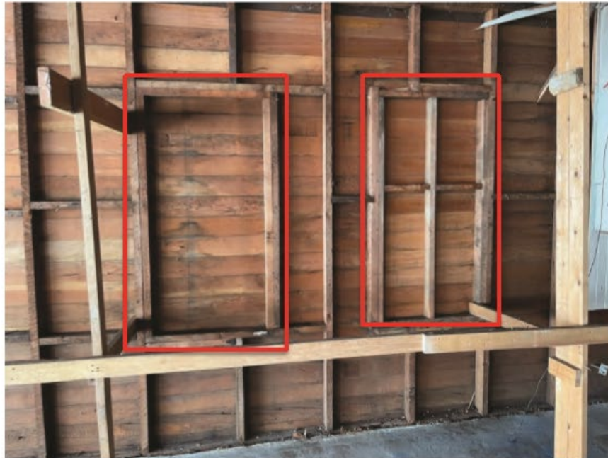
Figure 29a: Window openings on interior, west side wall: frames are intact, but boarded over with a siding profile identical to that in place elsewhere on that side.
