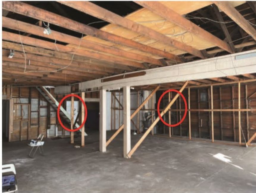
Figure 28: Exposed interior showing one original window still in place, painted white and on rear wall (left, circled above) and a single window frame on the east wall (right, circled above); magnified rear window, below.
