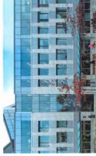
Capitol Park, office building, Victoria BC Appropriate window-to-wall ratio with punched windows and less curtain wall areas
