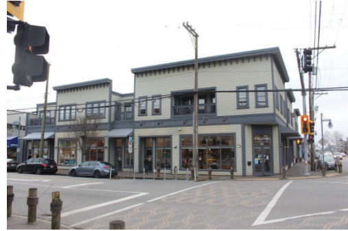
Parapet/cornice, cladding, façade articulation & window pattern
