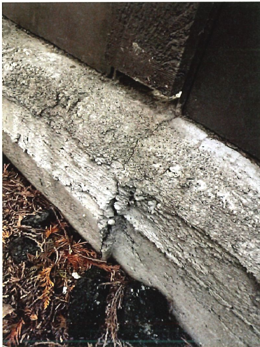
Photo 5 Cracks on CIP Concrete Retaining Wall
