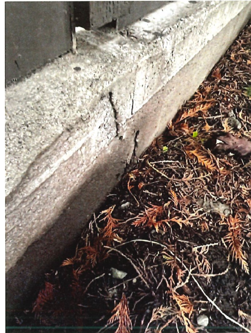
Photo 6 Cracks on CIP Concrete Retaining Wall
