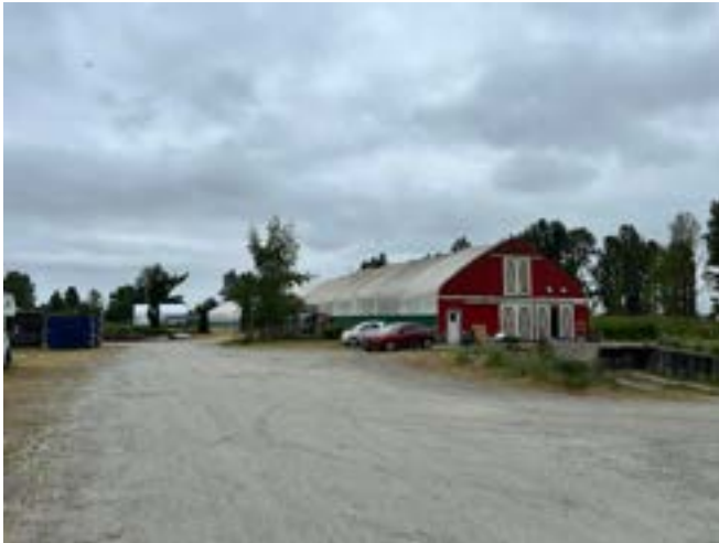
(a) Poultry barn quonset.
