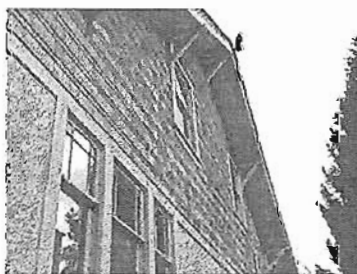
Shingle cladding at side gables
