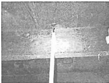
2x6 Main floor joists
