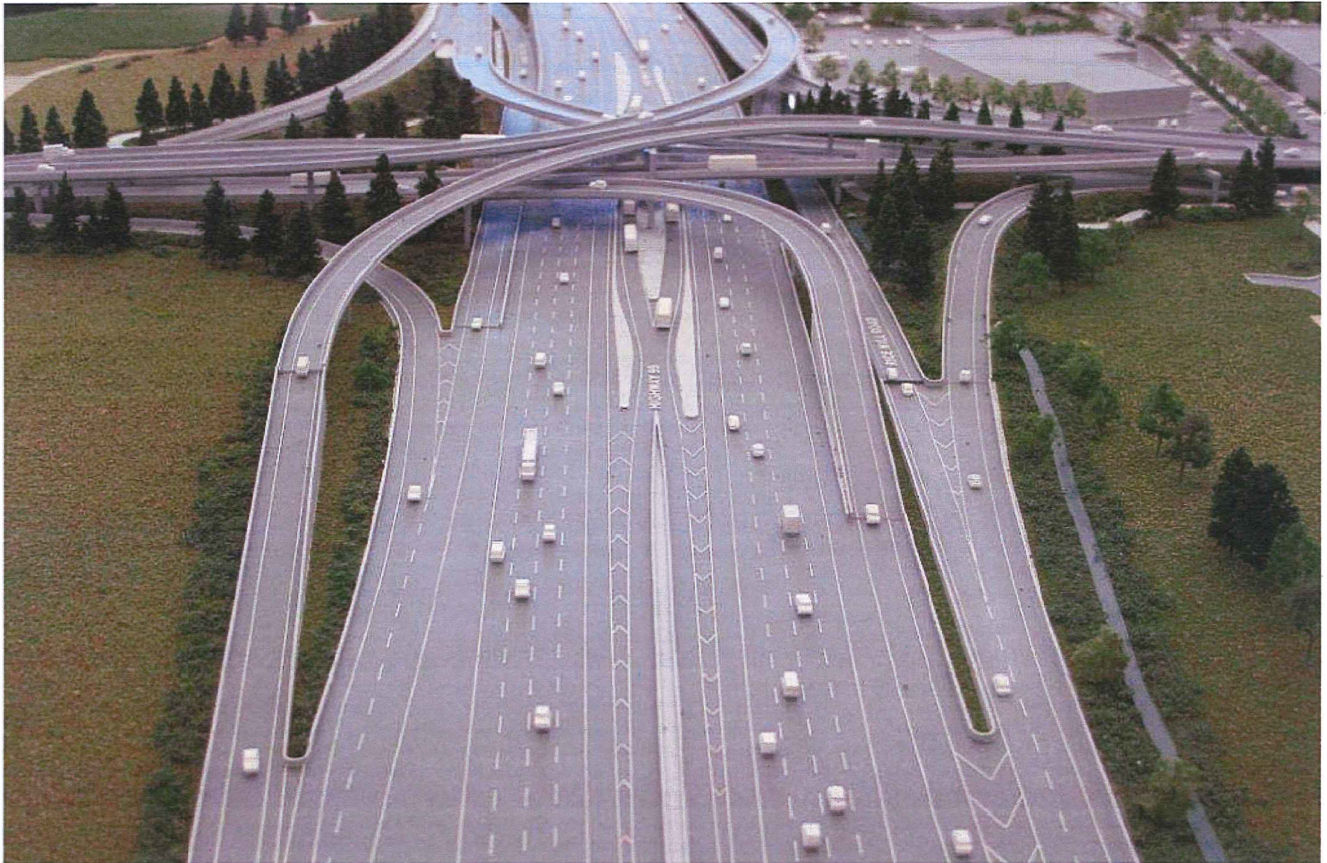
Facing south toward Steveston Highway Interchange
