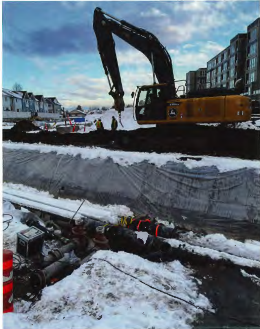
Implementing distribution piping in the ADEU.
