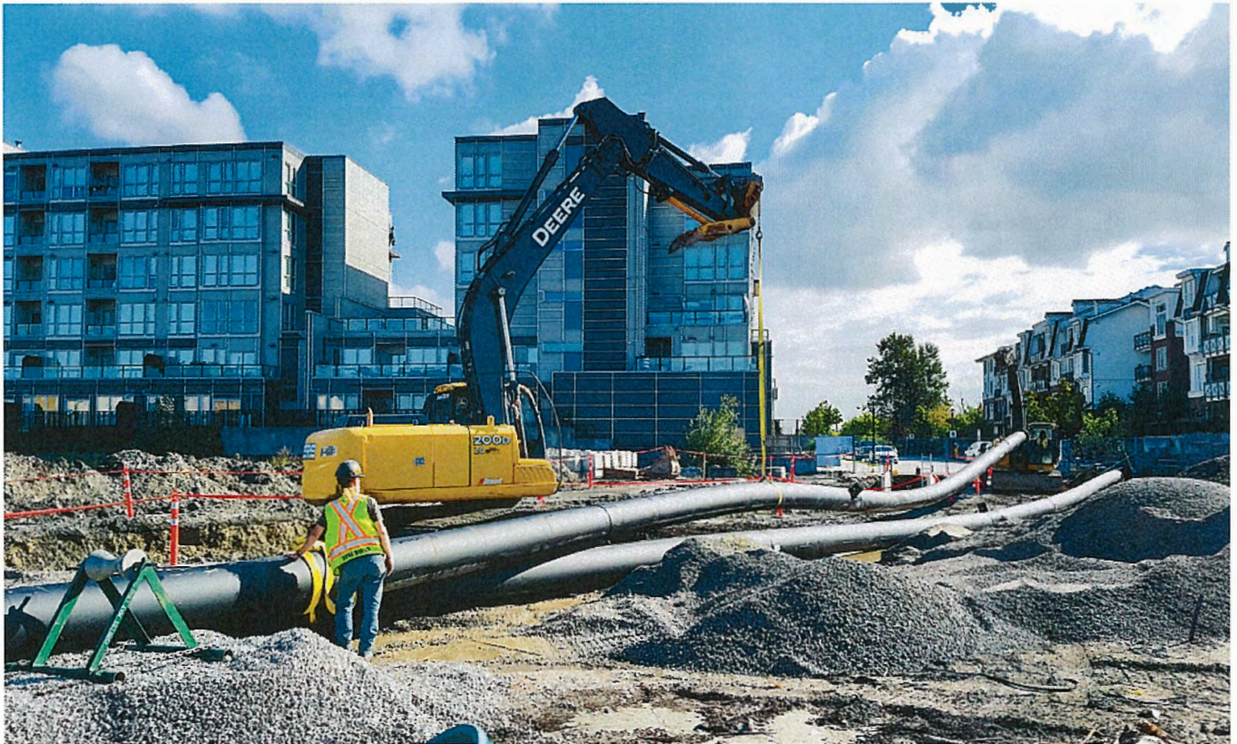
New distribution piping being installed in the Alexandra District Energy Utility service area to connect the Westmark and Berkeley House buildings
