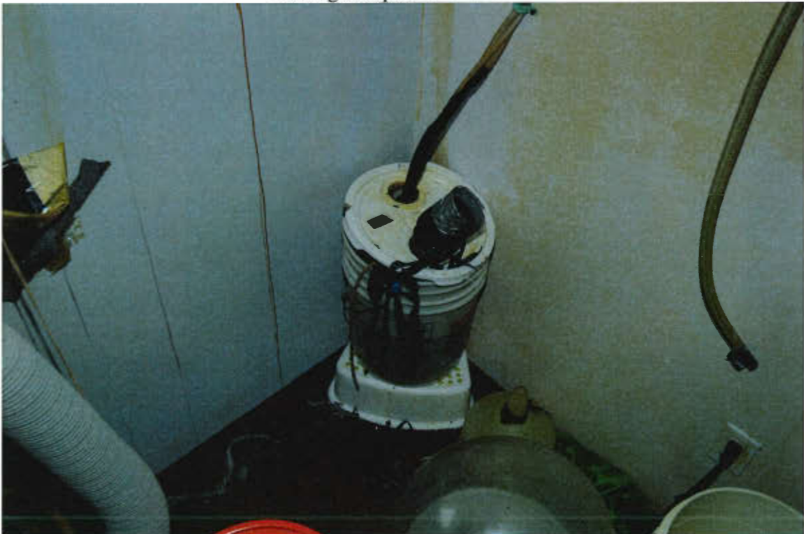
Image 9: Image of make shift vessel to store an unknown chemical. Note heavy staining on walls due to chemical residue
