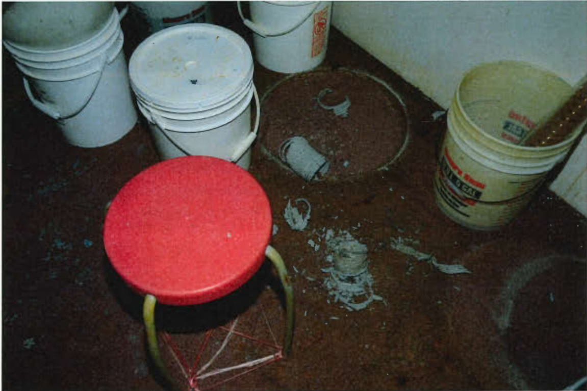
Image 8: various chemicals found in room, note heavy staining on carpet. Chemicals would have soaked through carpet and into floor studs.
