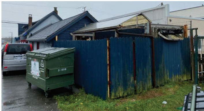
Rear of the building
