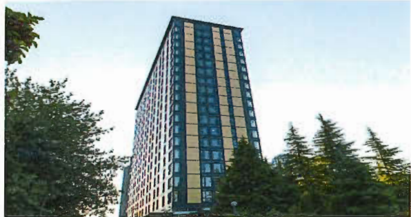
Figure 3: Brock Commons, UBC, in Vancouver, BC
