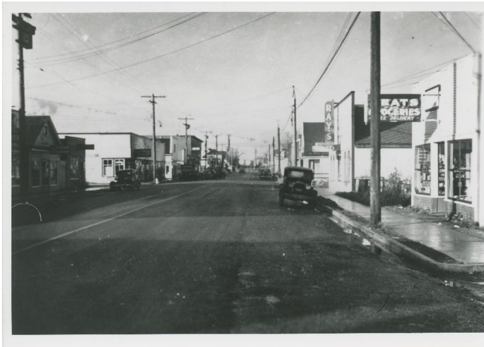
Moncton Street, 1949-54. 3871 Moncton Street is at far right of photograph. City of Richmond Archives, Raymond Owens Photograph # 1999 22 5.
