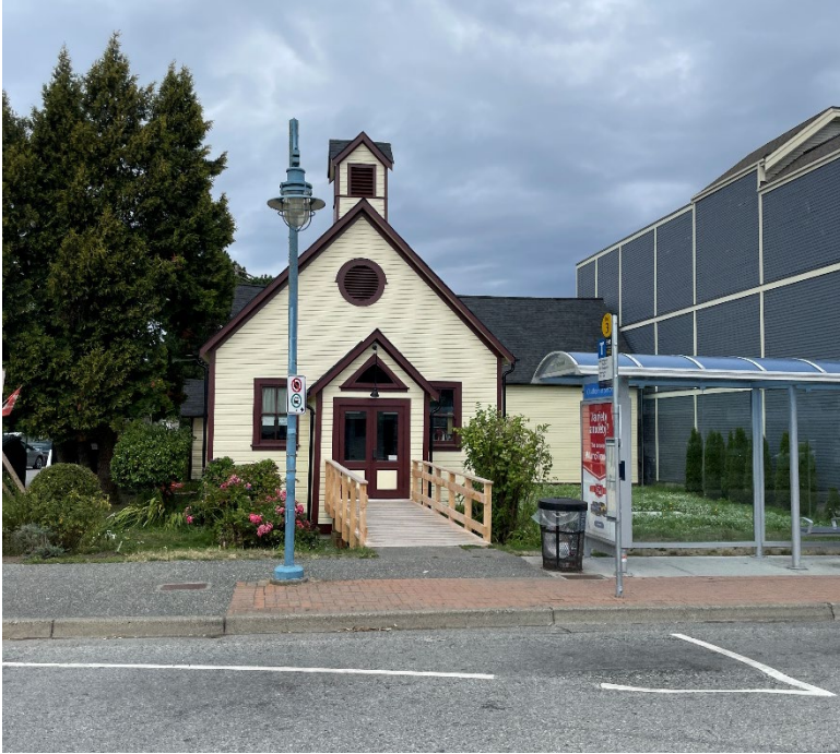
View from Chatham Street, September 2025
