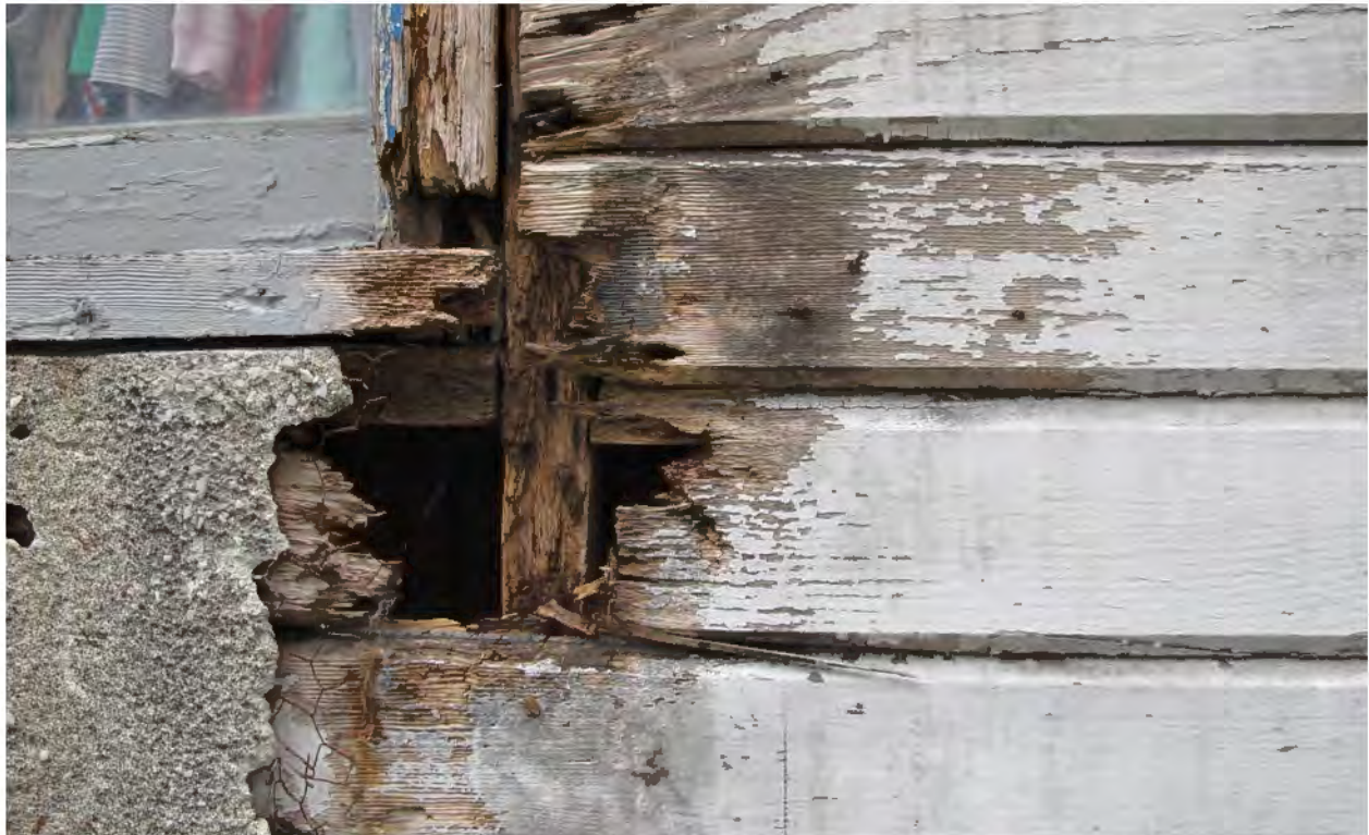
Above and below: Existing condition of exposed wooden drop siding, and dry rot condition at window corners.
