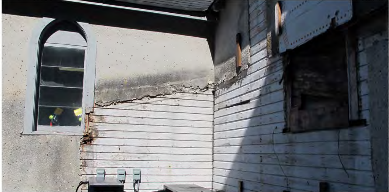
Above and below: Existing condition of exposed wooden drop siding, and dry rot condition at window corners.
