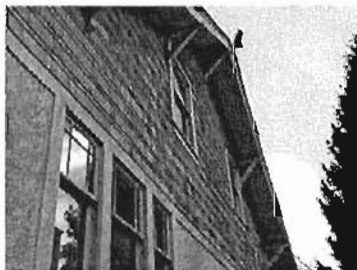
Shingle cladding at side gables
