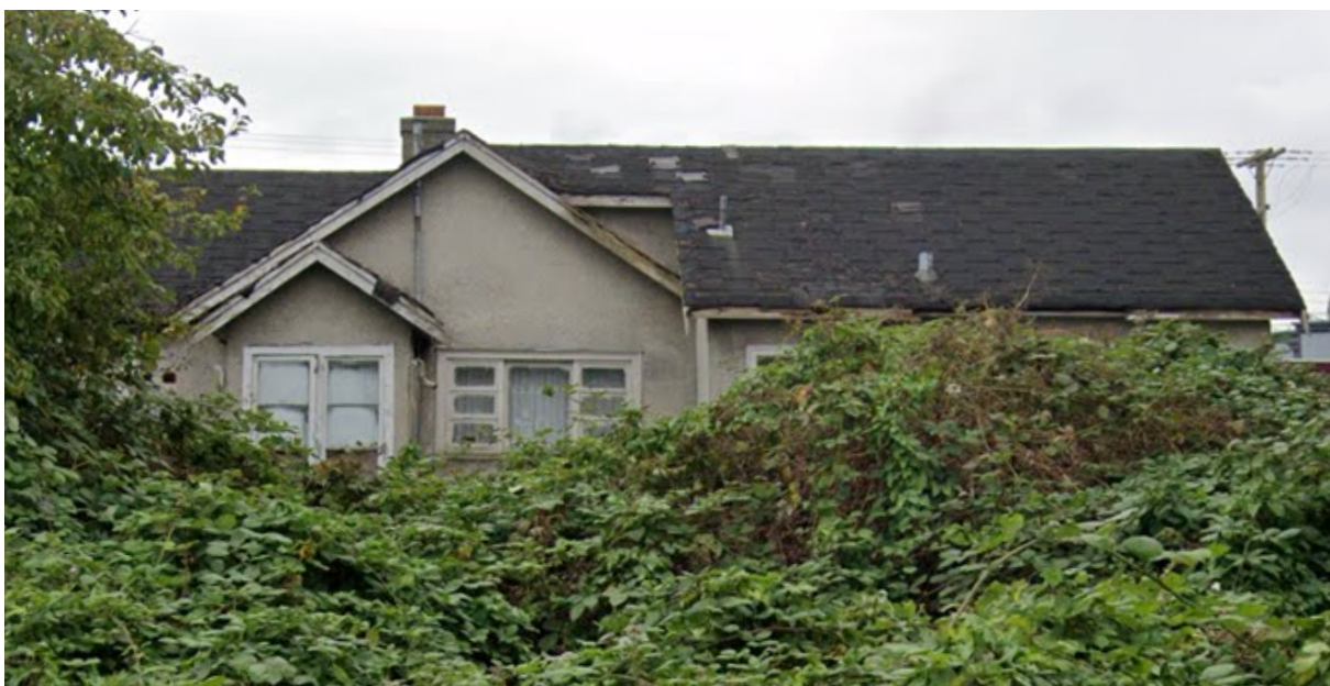
Figure 21: Subject site, limited rear face seen from the lane, illustrating the tripartite window arrangement with bold horizontal muntins on the flanking windows
