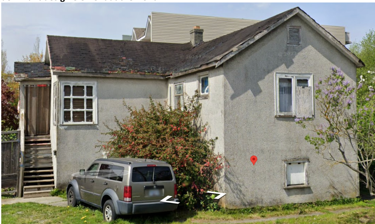
Figure 20: Subject site, seen from Second Avenue, illustrating the lack of other competing or dominant design elements on the exposed street sides of the house
