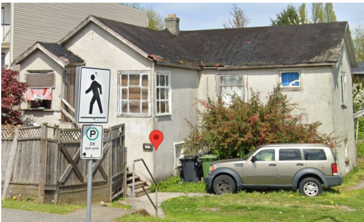
Figure 19: Subject site, illustrating the historic wrap-around (corner) window as the dominant design element at the front
