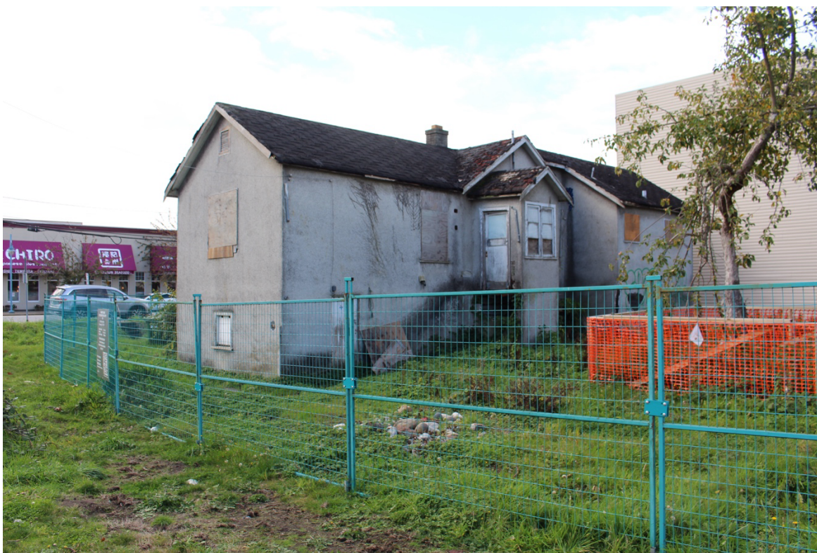
Figure 18: Subject site, house built in 1950 (rear).
