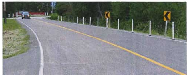
Anti-skid Surface & Delineators at No. 6 Road S-Curve
