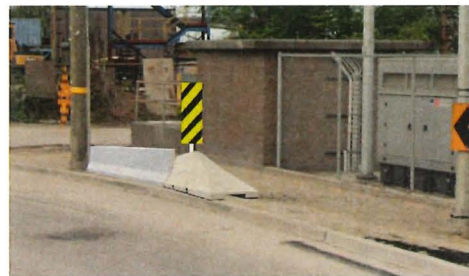
Figure 2: Example of Hydro Pole Protection at River Road and No. 6 Road
