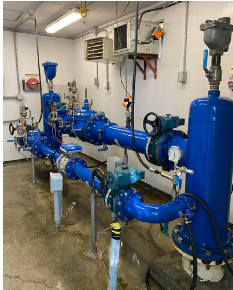
A look inside a pressure reducing valve station.
