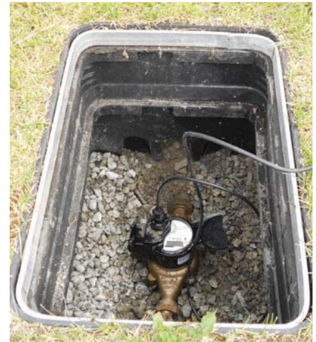
Installed water meter
