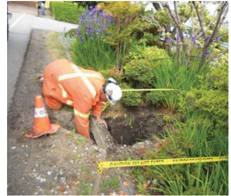
Water Meter Installation
