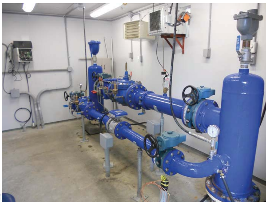
Inside the pressure-reducing valve station
