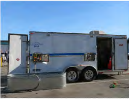
Emergency treatment trailer exterior
