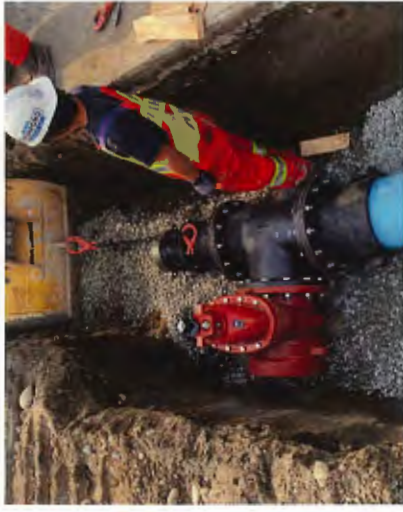
Staff helping an excavator line up a fitting during a watermain capital construction project.
