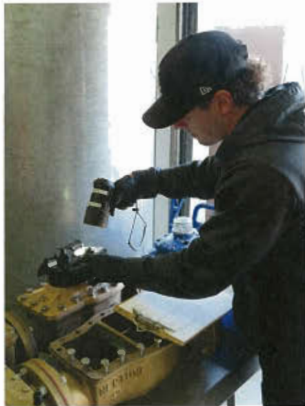
Water meter maintenance
