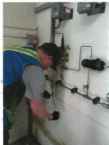
Taking a sample inside the PRV
