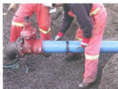
Installing a PVC pipe
