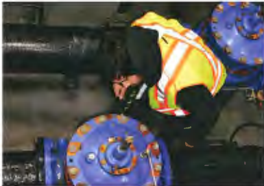
PRV station maintenance
