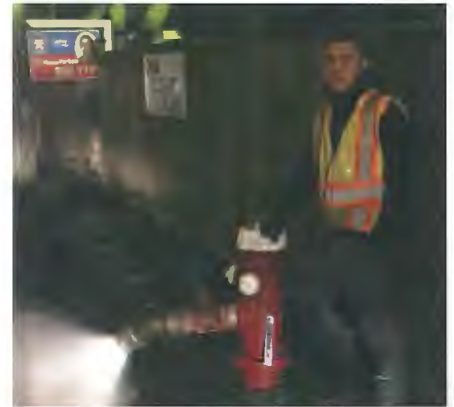
Flushing the watermain
