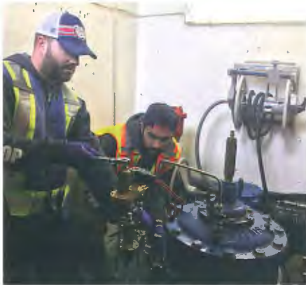
Pressure management system installation
