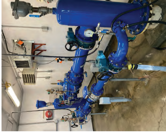
A look inside a pressure reducing valve station.
