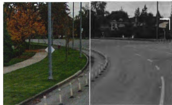
Figure 3: Shoulder Delineators at Railway and Granville
