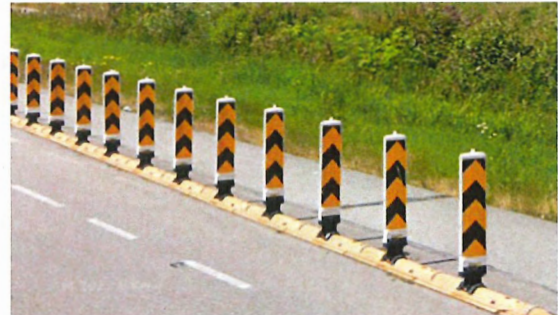
Figure 2: Curb-mounted Delineators at Garden City and Westminster
