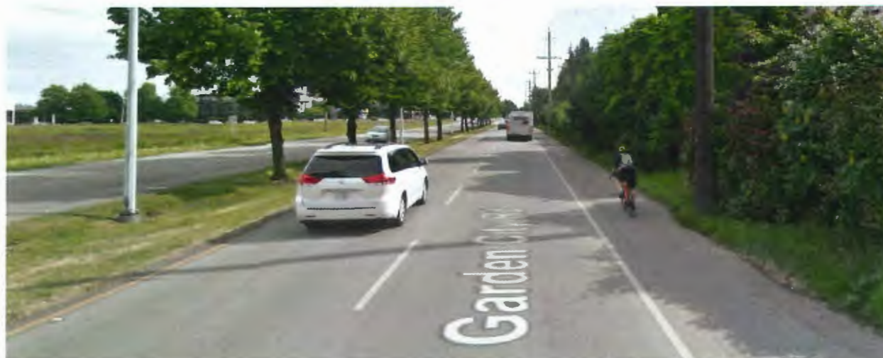
Figure 1: Existing Condition on Southbound Garden City Road south of Lansdowne Road
