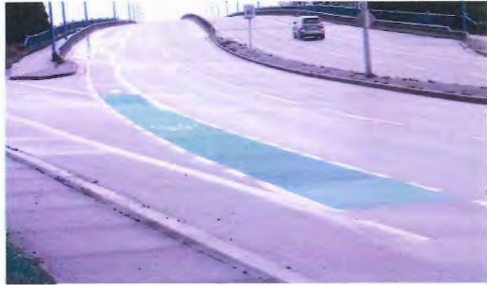
Figure 2: Green Surface in No. 2 Road Bike Lane
