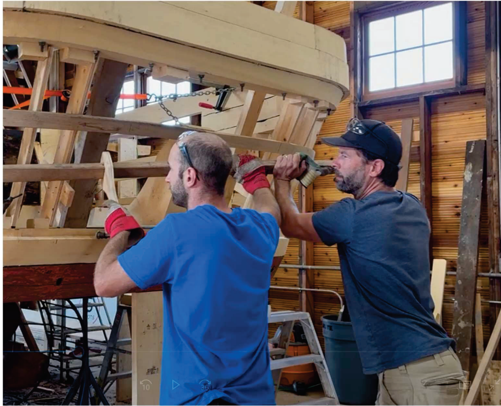
Shipyard Operations Supervisor and Shipwright Assistant installing steam-bent members on Crystal S , 2025
