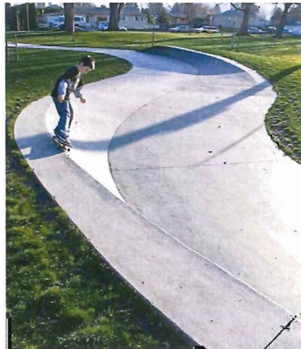
CONCRETE WAVE TO DIRECT DRAINAGE
