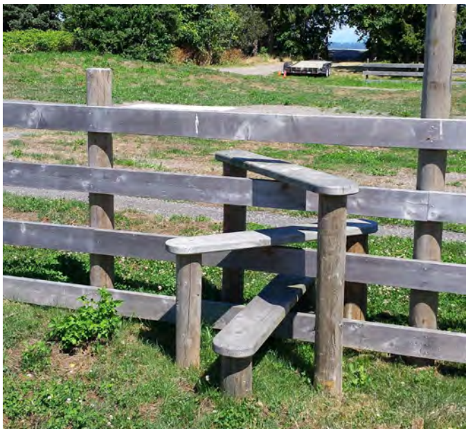
A fence stile integrated into the paddock fence at Terra Nova Adventure Play Environment.
