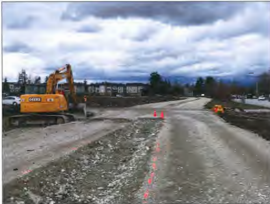
Above: Substantially complete portion of bicycle and pedestrian paths along No. 4 Road. Final top layer of fine gravel not yet installed.
