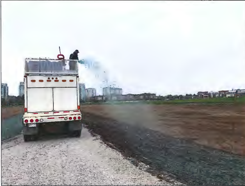
Above: Hydroseeding equipment applying native grass seed mixture to exposed soil slopes along farm access road.
