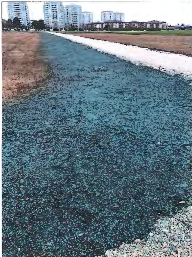
Above: Previously exposed soil after hydroseeding application.
