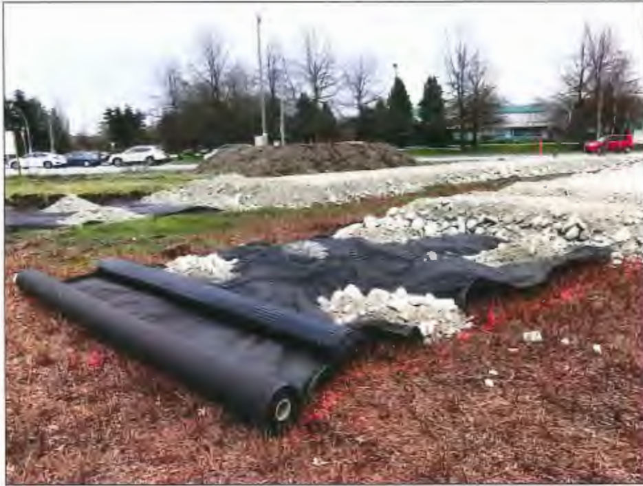
Above: Initial stages of perimeter path construction (geotextiles and crushed stone base layer) along No. 4 Road.
