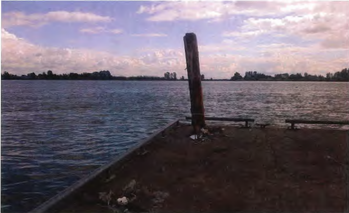
Figure H Deadhead puncturing through the bottom of a concrete float in Richmond along the Fraser River (source: City of Richmond).
