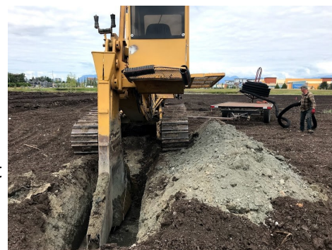
Drain tile installation, June 2018
