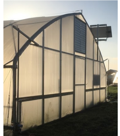
A wire above the peak of each high tunnel discourages bird perching.
