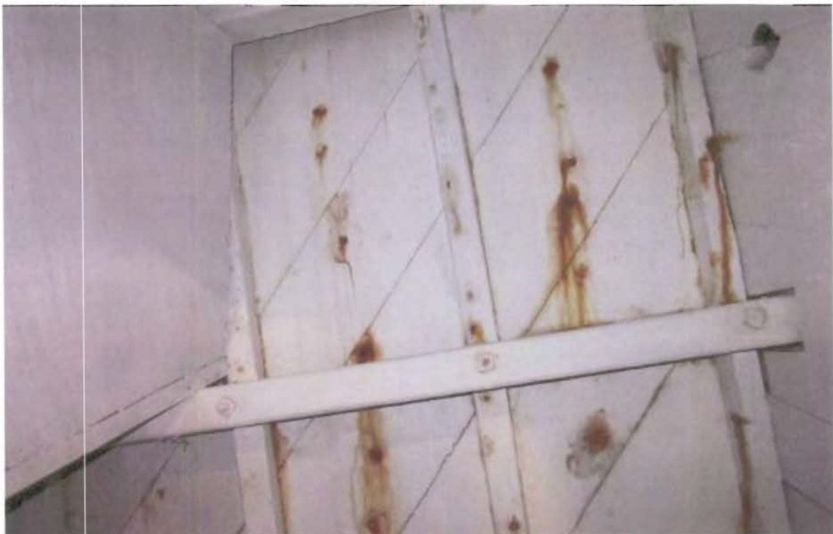
Photo #10 Detail of corroded fasteners inner planking
