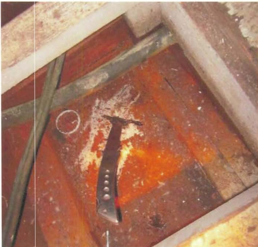
Photo #8 Deterioration of inner planking
