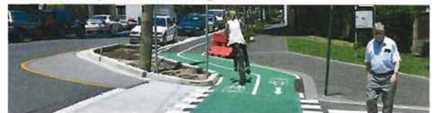
Temporarily paint and mark existing crossing with "elephant's feet" indicating the crossing is shared for pedestrians and cyclists.
