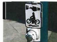
Button signal at appropriate height for cyclists.
