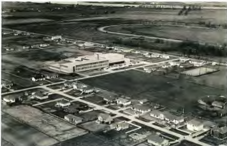
Brighthouse aerial view, 1953
