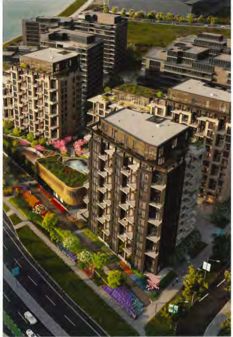
Aerial perspective of the site from the Southwest
