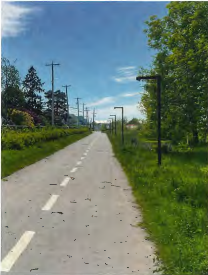
Example of pedestrian scale pole lights along multi-use path on Sea Island (photo credit: City of Richmond)
