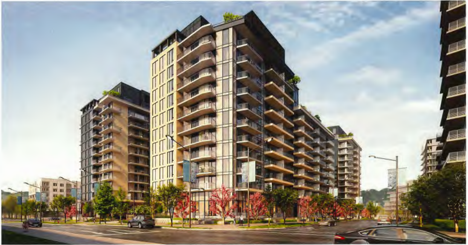
Street level view of the development facing Northwest
