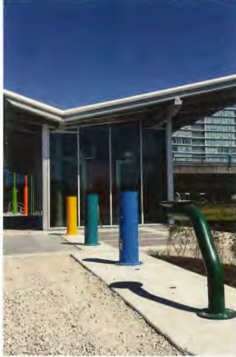
Germaine Koh, No. 2 Road North Drainage Pump Station , 2018. Richmond, BC
