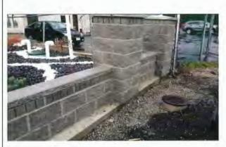
January 24, 2020 – Rim of inspection chamber located above surrounding ground elevation
